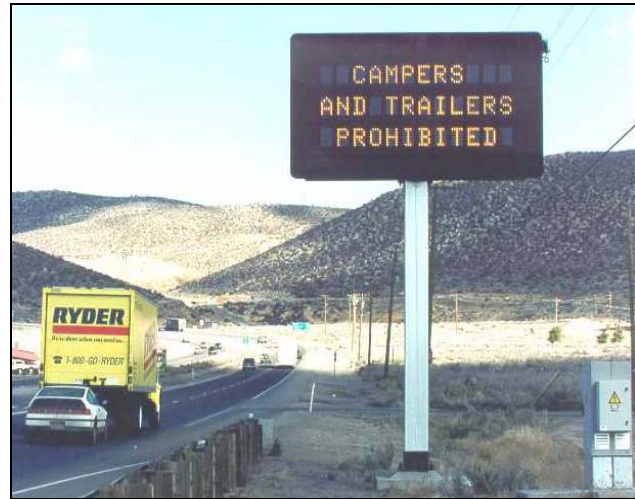
Nevada DOT High Wind Warning on DMS
