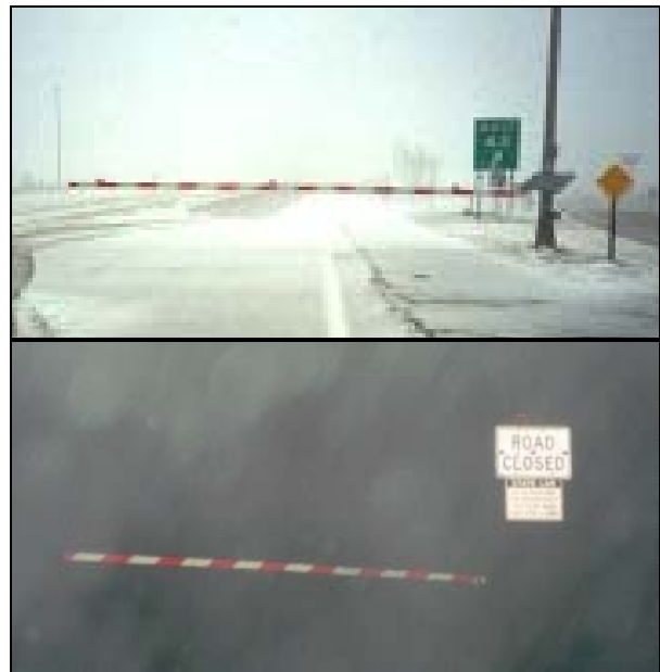
Minnesota DOT Ramp Gates and Warning Signs
